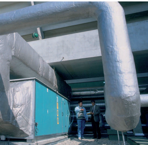
Circulating pumps for building management
